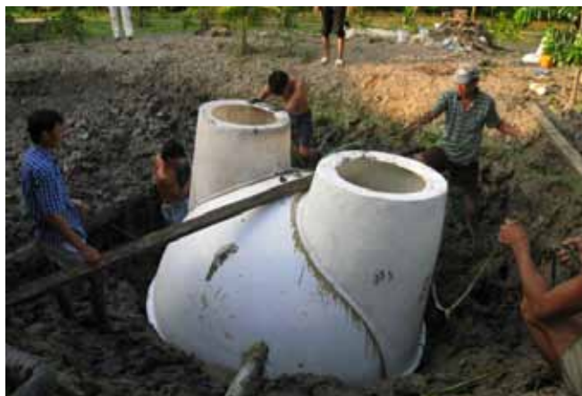
Installing a household biogas digester Photo courtesy: Le Thi Thoa
