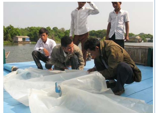
Investigating Preliminary Floating Biodigester Design
